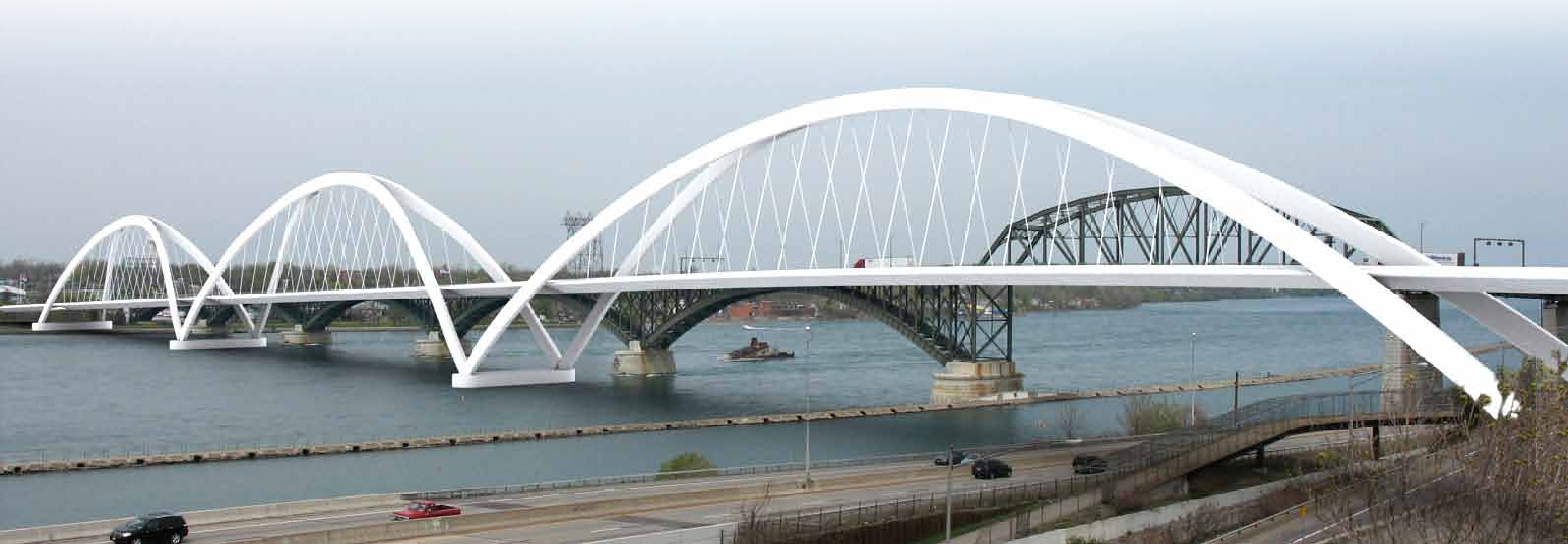
Three Span Arch Signature Bridge Concept
